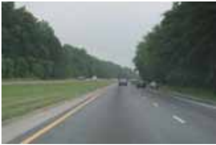
Figure 4-28: On the Baltimore-Washington Parkway turf shoulders are reinforced with a “dirty-stone” mix of soil and aggregate making it possible for turf to get established; Cars can easily move out of the travelway over the mountable curbs
