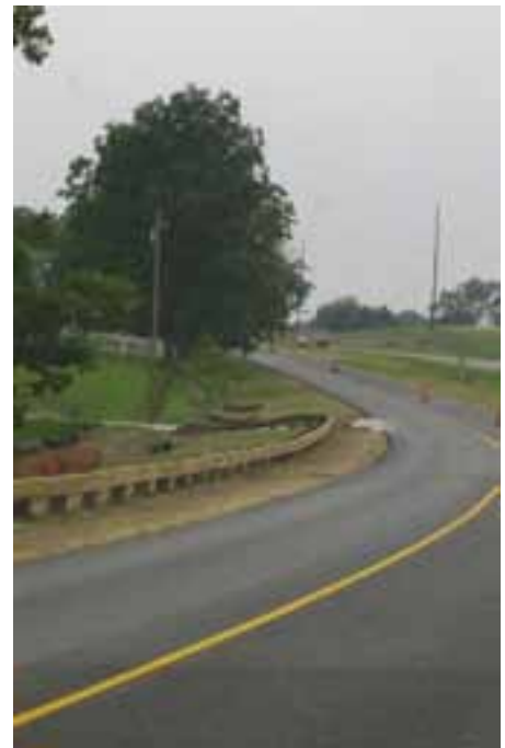
Figure 4-26: Steel-backed timber guardrail on Paris Pike (photo courtesy of HW Lochner)
