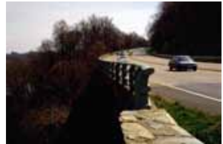
Figure 4-34: Bridge railing using tubular steel along the George Washington Parkway in Virginia
