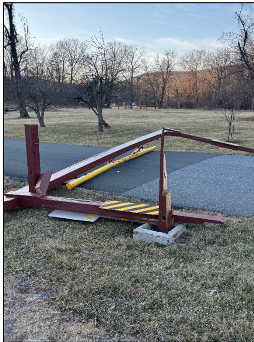
The damaged warning portal.
