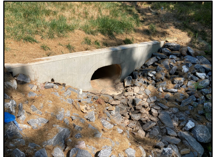
End of Channel Facing Culvert
