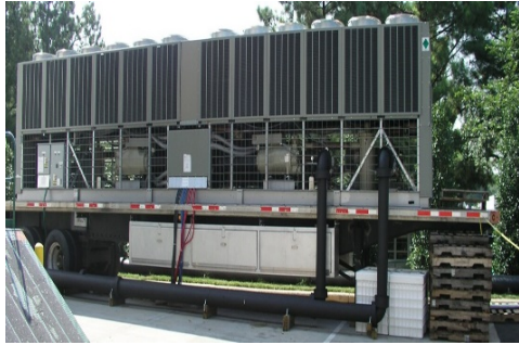
500 Ton Air Cooled Chiller up to 105 dB
