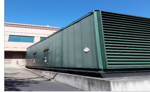
2 MW Generator up to 126 dB
