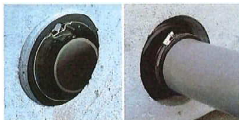
Example of appropriate pipe connection using a Kor-N-Seal. Note that the pipe connector does not protrude past the structures inside wall.
