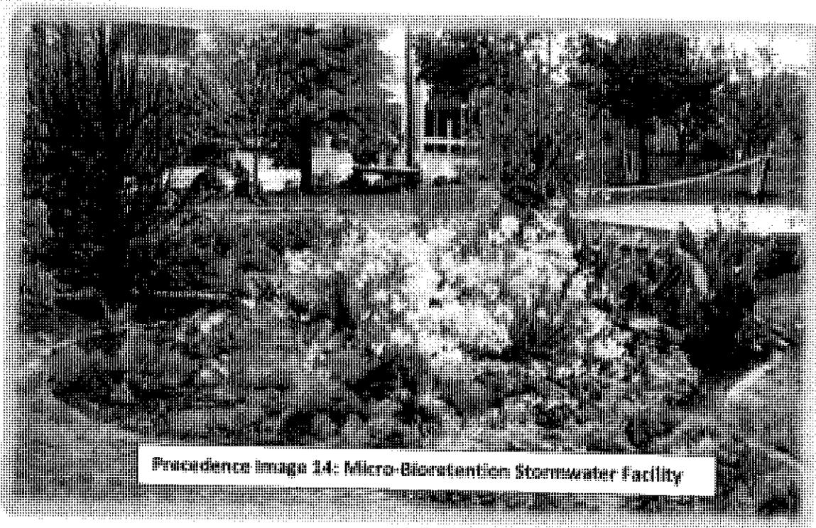
Precedence Image 3.4: Micro-Bioretention Stormwater Facility
