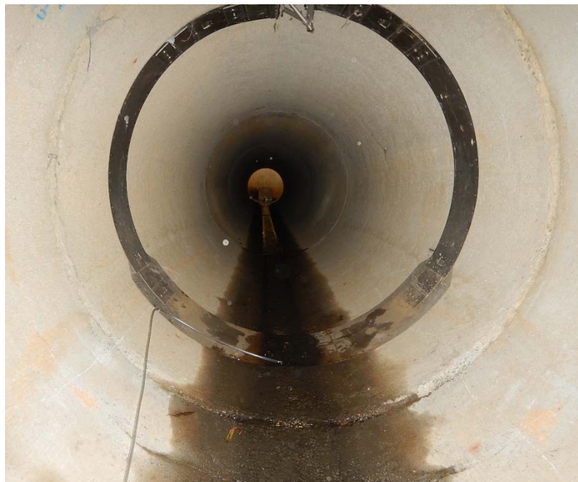
Figure 2-2b. Bubbler flow module located at the midpoint of the Pond-R outfall pipe sampling stage data for the Pond-R station.
