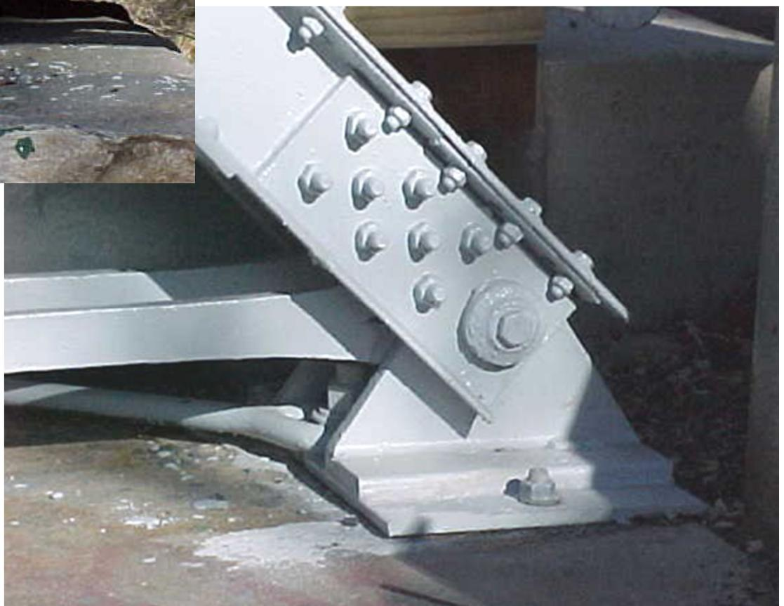
New fixed bearing at the southeast truss endpost.
