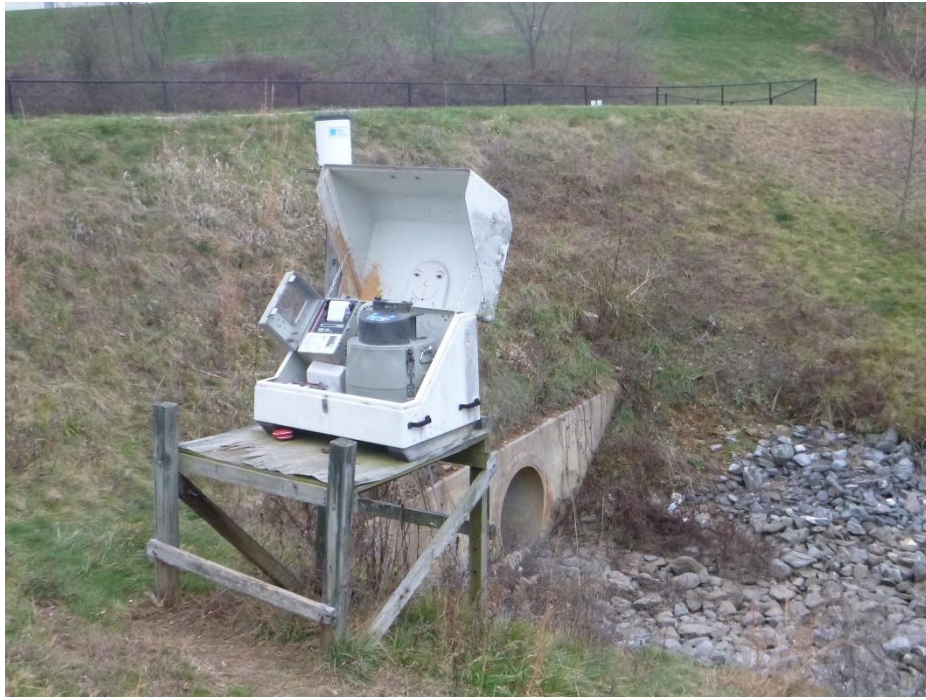
Figure 2-2. Villages of Urbana “Pond R” outfall water chemistry monitoring station and rain gauge. Photograph taken December 2015.
