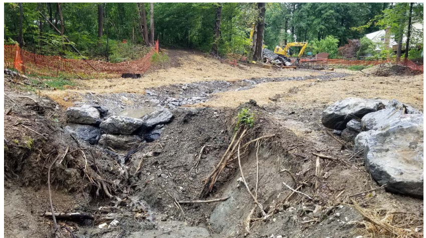
Raising the stream bed back to its original elevation at the Point of Rocks Stream Restoration Project
