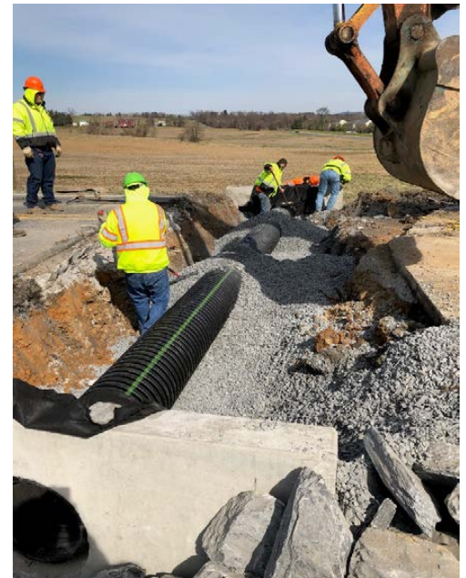
Installing a high density polyethylene drainage pipe and headwall under Ballenger Creek Pike
