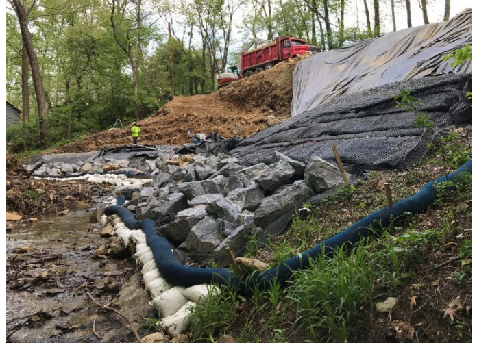
Slope stabilization on Mount Zion Road (Highway Network Systemic-General)
