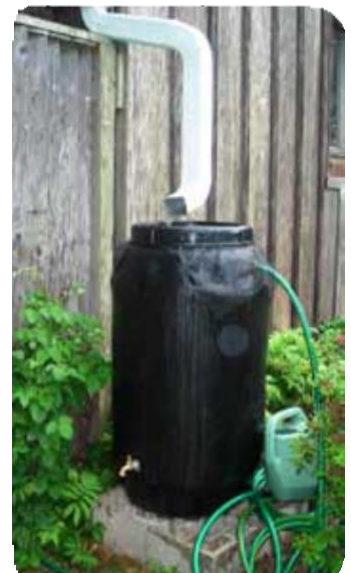
The screen on this rain barrel keeps out mosquitoes and minimizes drowning risk.
