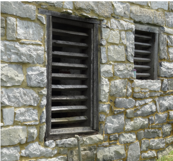
Wood louvers in a stone bank barn in Frederick County. Photo by Gary D. Baker, RA.
