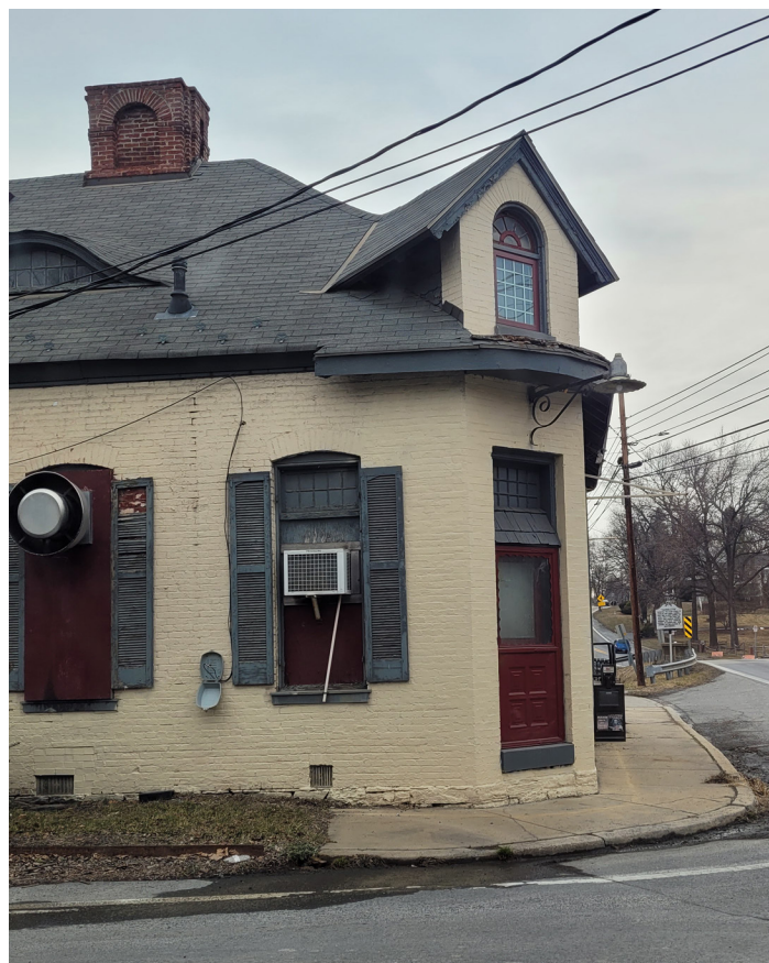
It is not recommended to modify window openings to accommodate the installation of equipment, particularly on a highly visible facade. Image by authors.
