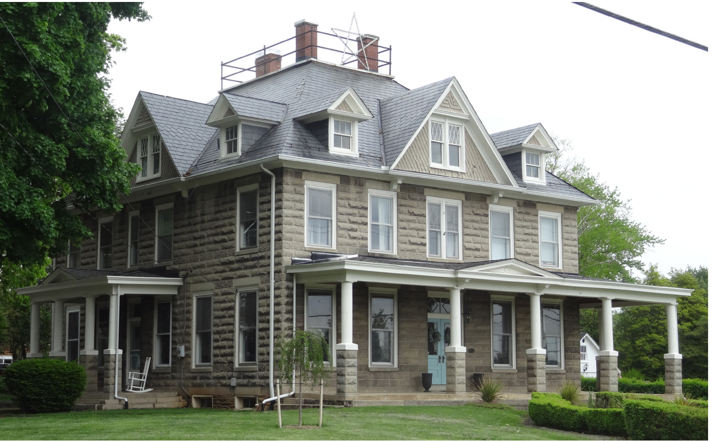
This house in Middletown has rusticated concrete block walls. Photo by Gary D. Baker, RA.
