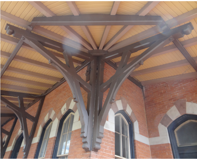
Point of Rocks Railroad Station structural framework supporting ceiling of protective overhang. Photo by Gary D. Baker, RA.
