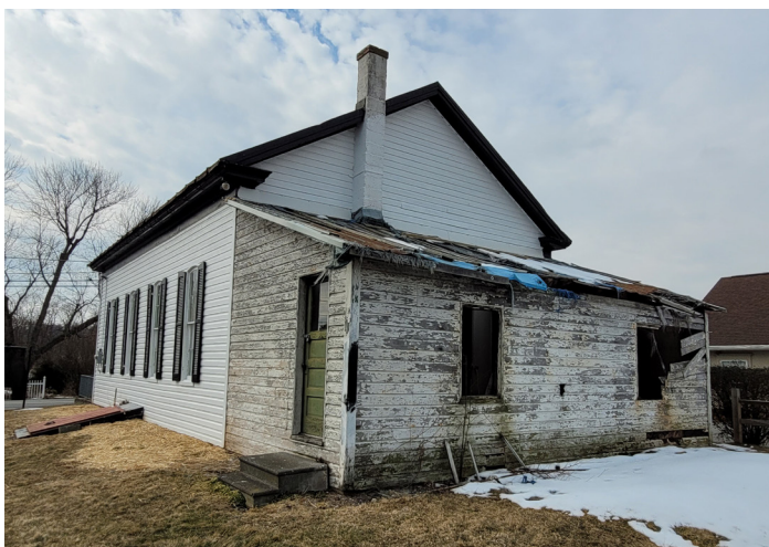
This shed roof rear wing was an early addition to the Rocky Springs Chapel near Frederick. It uses the same materials as the original and is well sited at the rear of the building. Photo by authors.
