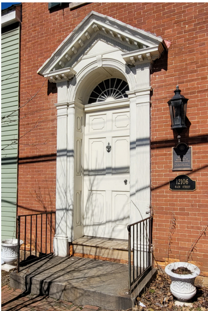
The pedimented entryway of the Abraham Jones House in Libertown has a paneled wood door with fanlight above. Photo by authors.
