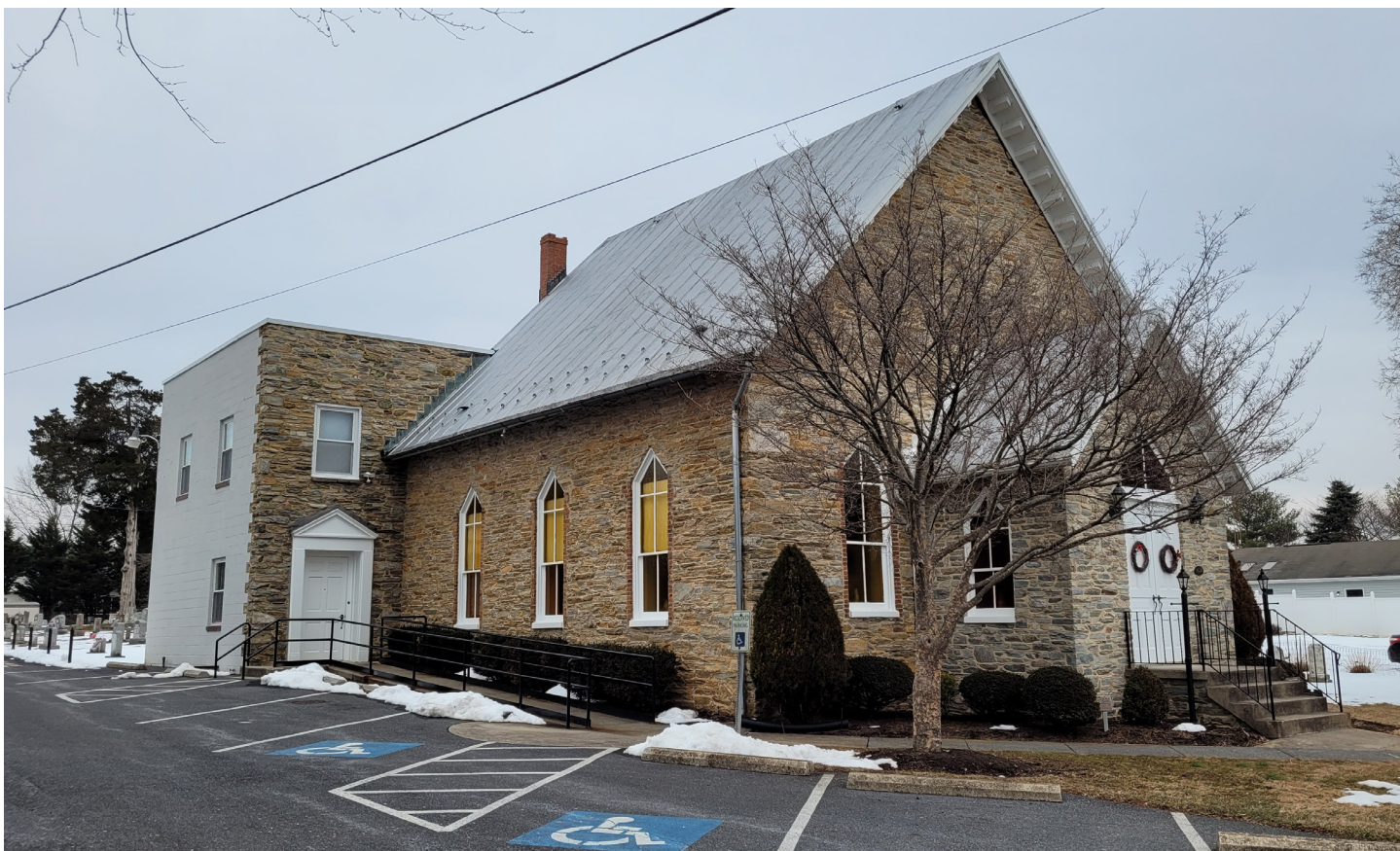
An accessible ramp and entry door was added to the Methodist Episcopal Church in Jefferson at the modern flat-roofed addition on the west side in order to keep the historic fabric of the original church entrance intact. Photo by authors.
