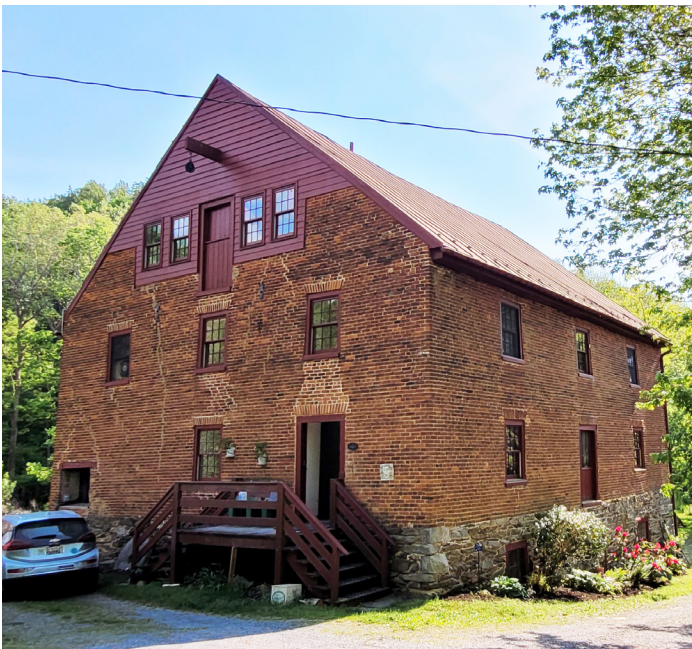
Common bond brick of the Lewis Mill, Jefferson. Photo by authors.
