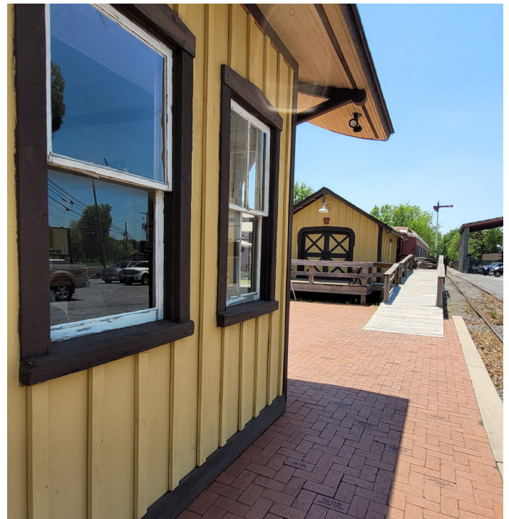
The Walkersville Railroad Station and Tool House have vertical board and batten wood siding. Photo by authors.
