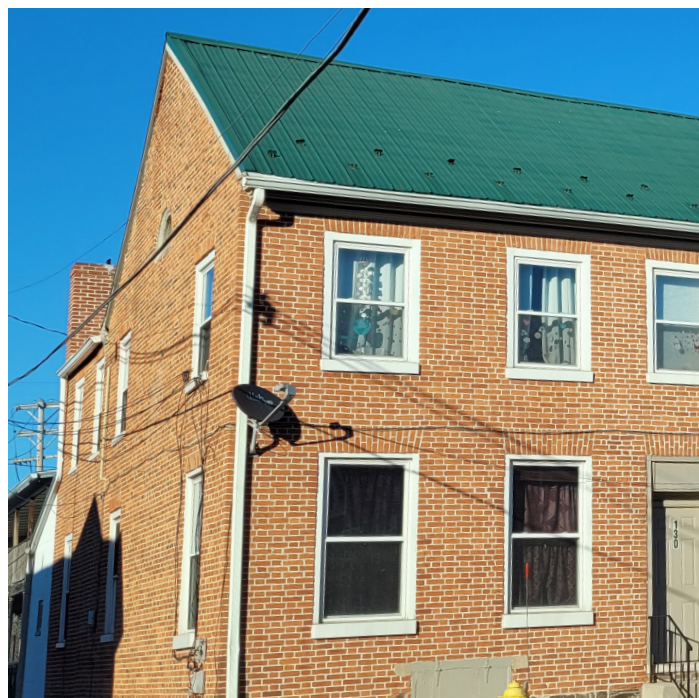
It is not recommended to mount equipment in conspicuous locations like this cable dish. Photo by authors.
