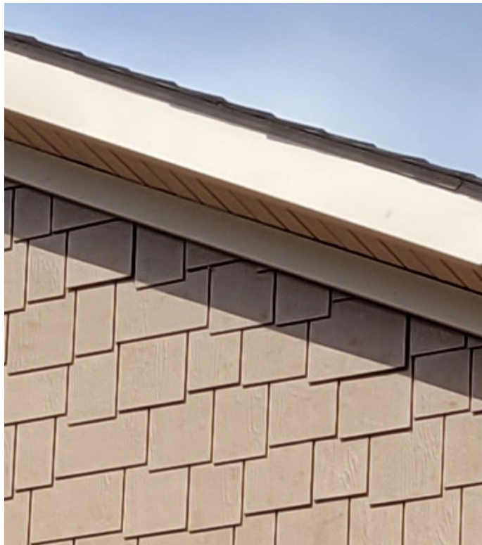
Example of a synthetic material (left) that is not an acceptable alternative for the traditional material. The synthetic shingles are too thin and flat to achieve the same profile and depth of the original. Photos by authors.
