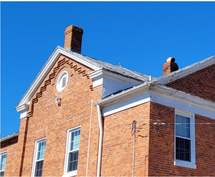
This church building in Libertytown has brick laid in Common Bond and corbelled brick at the cornice line of the gable. Photo by authors.
