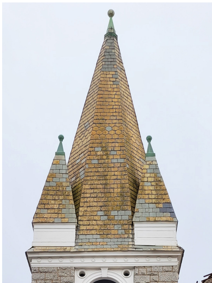
The belltower of the Buckeystown United Methodist Church is topped with a unique five pointed slate spire. The large central spire is hexagonal and the four corner spires are pyramidal. Each is topped with a finial. Photo by authors.
