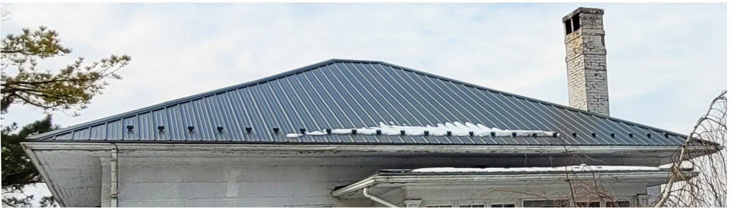
This modern metal roof has crimped, narrow panels and does not match the detailing found on an historic metal roof. Photo by authors.
