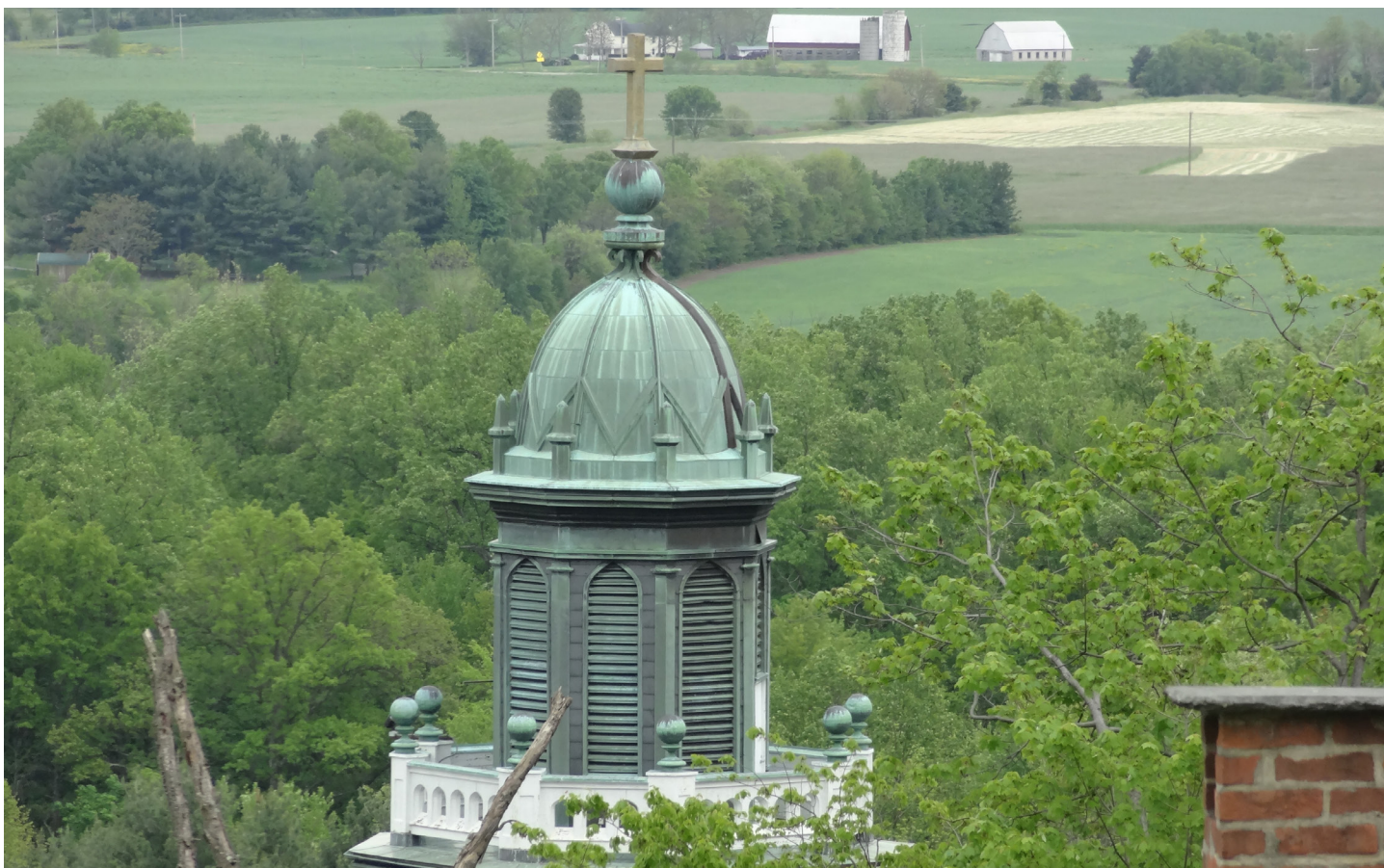
Copper-clad cupola at Mount Saint Mary's Seminary in Emmitsburg. Photo by Gary D. Baker, RA.
