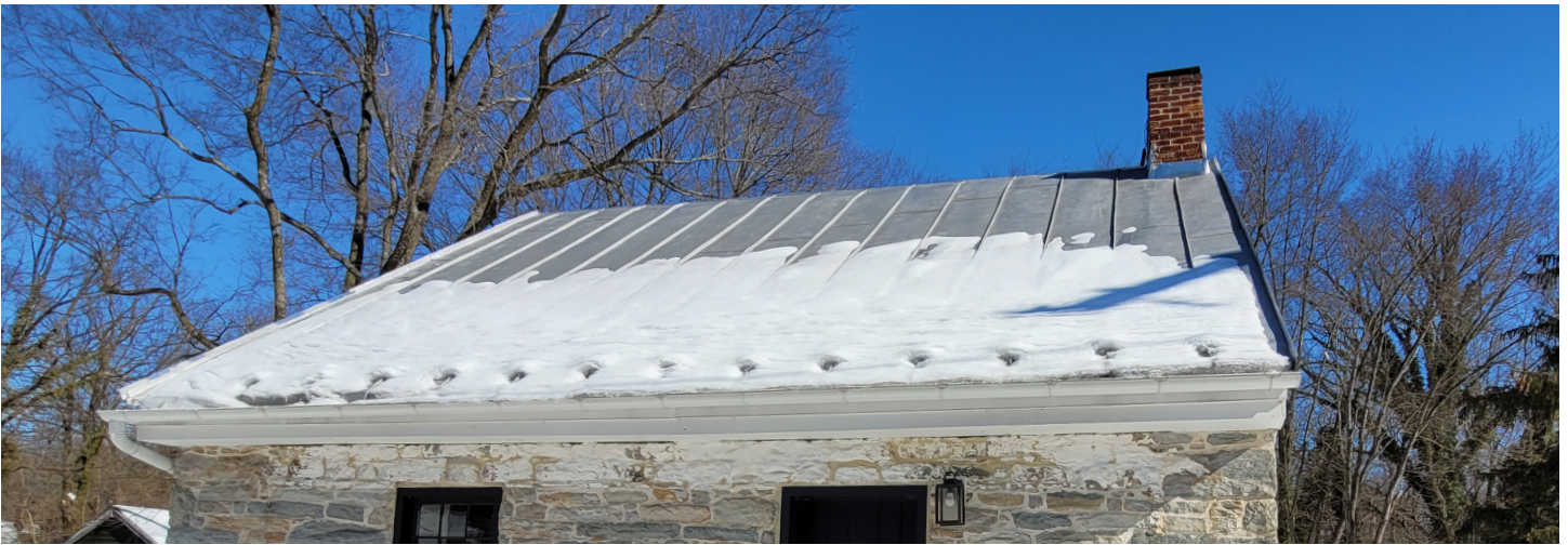
Standing seam metal roof of the Forges House in Catoclin Furnace; notice the spacing of the seams and profile of the panels. Photo by authors.
