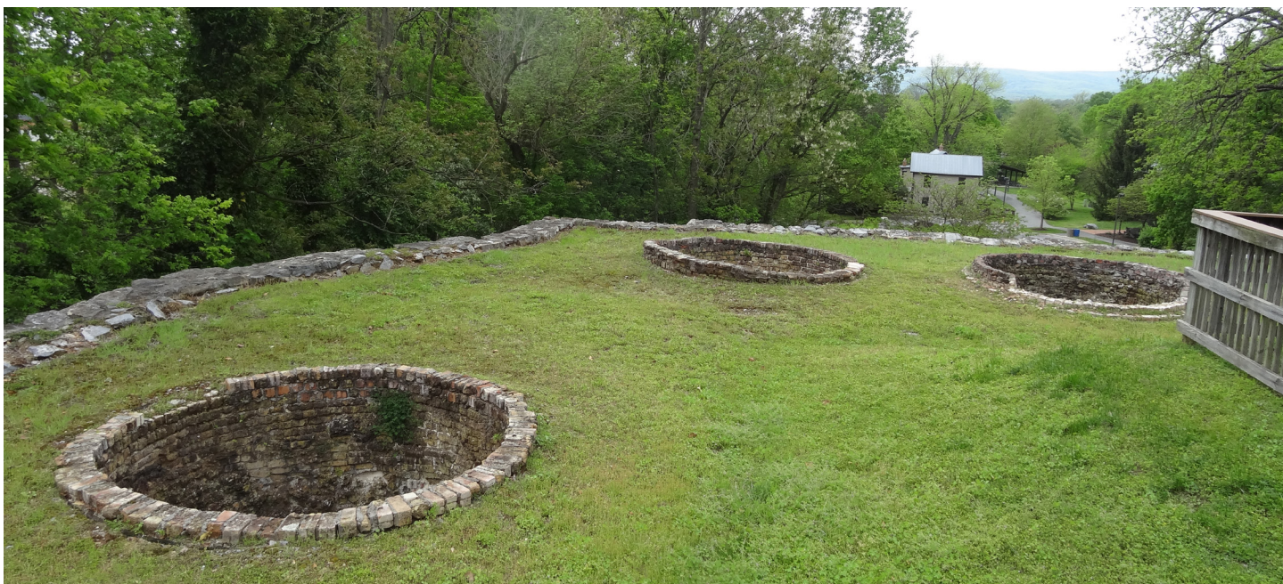
Tops of lime kilns where raw limestone was dumped to be heated to produce powdered lime at Fountain Rock Park and Nature Center in Walkersville. Photo by Gary D. Baker, RA.
