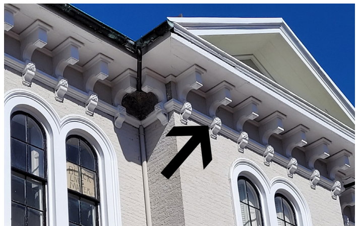
The cornice of Tyson Mansion on E. Church Street in Frederick has decorative brackets. Photo by authors.
