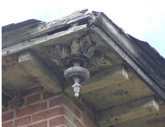
Deteriorating wooden pendant at the Point of Rocks Train Station. Photo by Gary D. Baker, RA.
