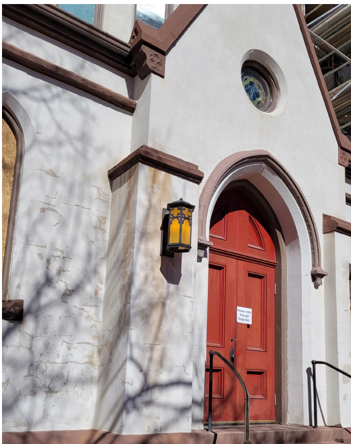
The Evangelical Lutheran Church in Frederick is made of brick walls covered in stucco. Photo by authors.
