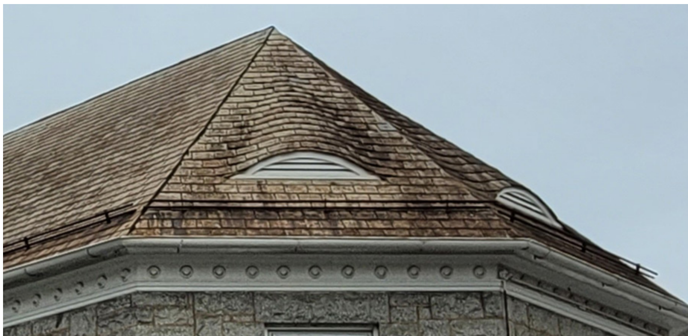
The louvers to vent the roof of Buckeystown United Methodist Church, Buckeystown, are set in small brow dormers. Photo by authors.
