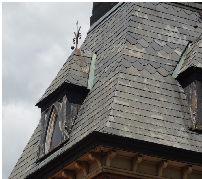
The slate roof at the Point of Rocks Train Station has dormer windows topped with finials. Photo by Gary D. Baker, RA.
