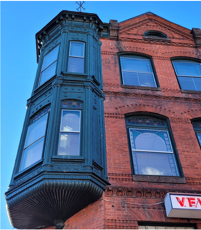
The storm windows on this building in Emmitsburg have narrow frames that align with the meeting rails of the windows, but should be painted a dark color to match the window frames. Photo by authors.
