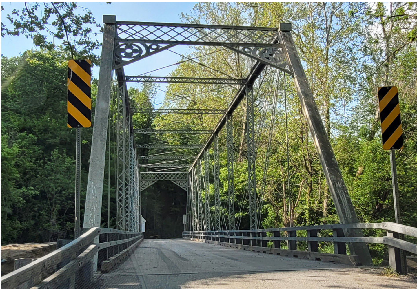
The Poffenberger Road Bridge near Middletown is an example of a Whipple thru truss iron bridge. Poffenberger Road is a designated Frederick County Rural Road and one of the few gravel roads that includes a metal truss bridge. Photo by authors.
