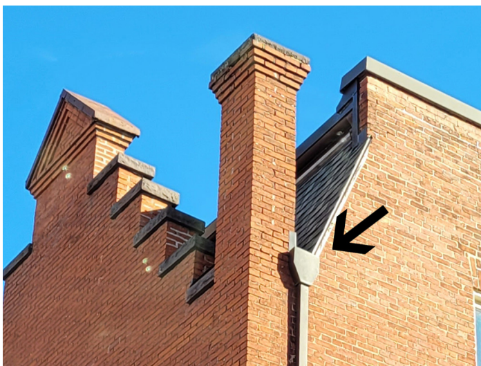
The gutters are concealed behind the brick parapet of the Sovran Bank Building in Thurmont. Photo by authors.
